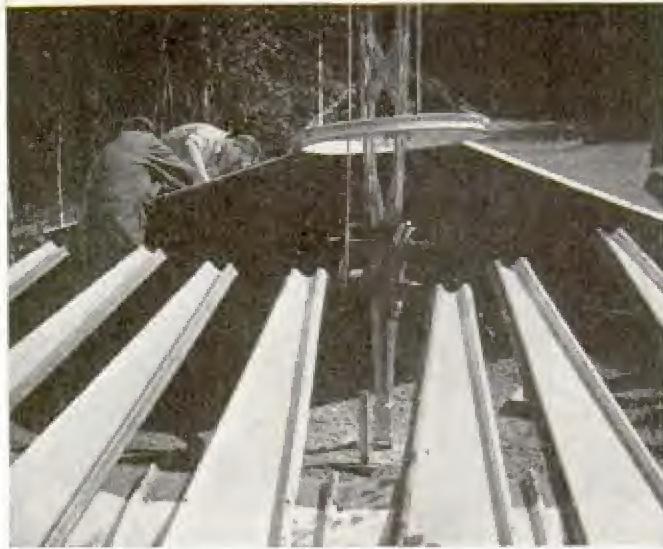
Erecting the circular house starts with the roof, made of metal sheets and dome shaped, which is assembled on the ground (below). It is hoisted to position up a mast
